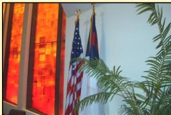
There are 12 windows each with three panels. All the colored glass was cut and bonded with a clear sealant. The lower panels of all windows have two layers of colored glass on the inside and one layer on the outside. The lower panels are translucent but not transparent, thereby affording privacy at eye level.
